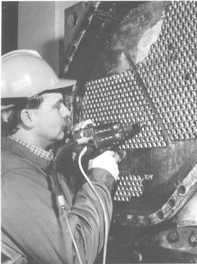
Eddy current examination of a heat exchanger.
