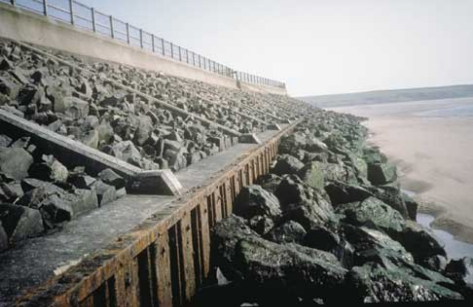
Rock faced concrete revetment
