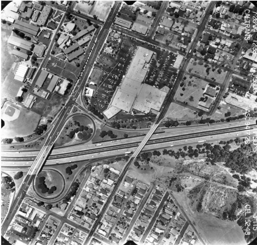
Figure 1. 1:3000 Aerial Photograph (Reduced to 85%)
