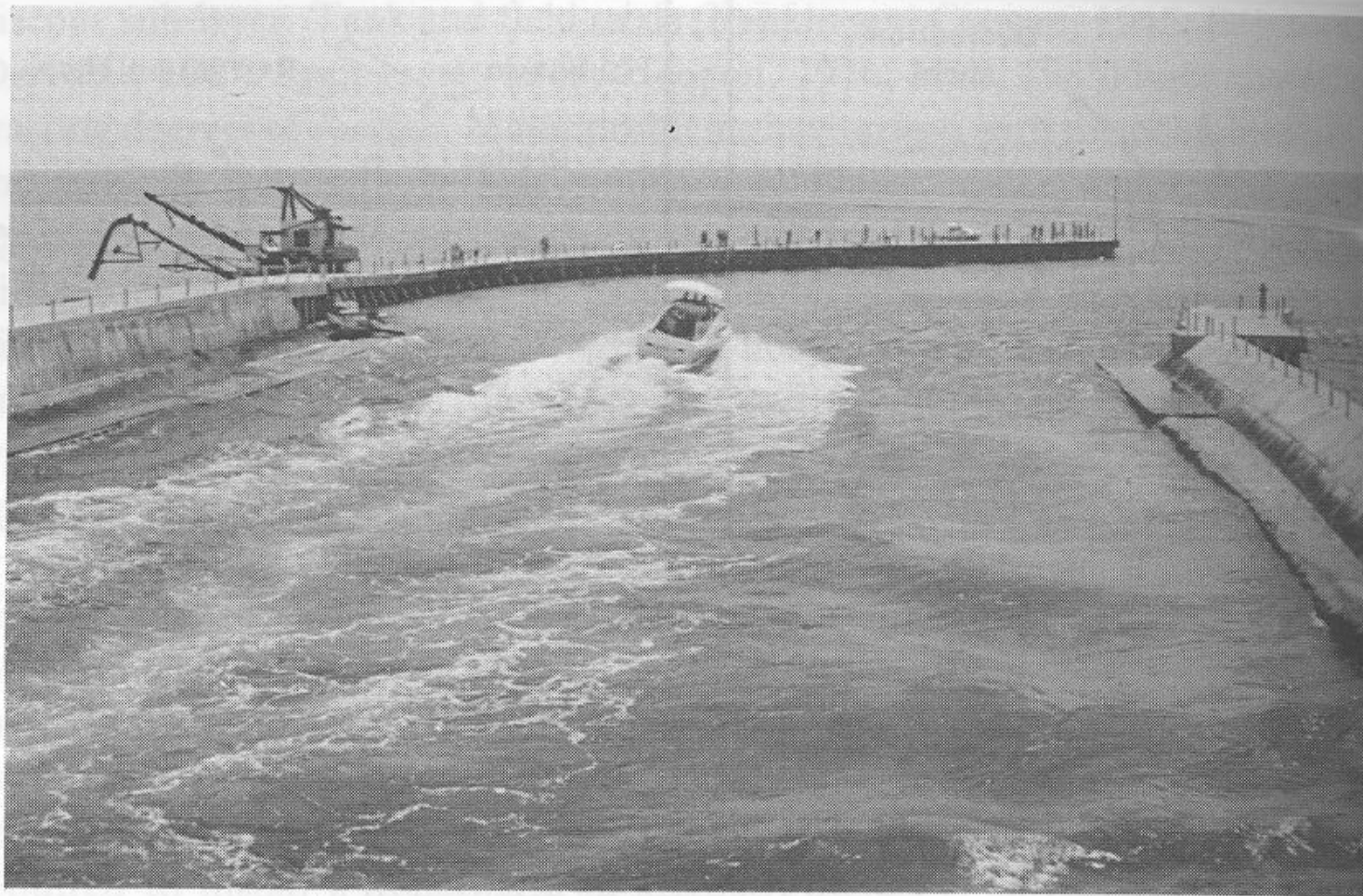
Figure 230. South Lake Worth Inlet by-passing plant in 1977. Sand from the updrift (northern side) is pumped across the inlet and redeposited on the downdrift side.
