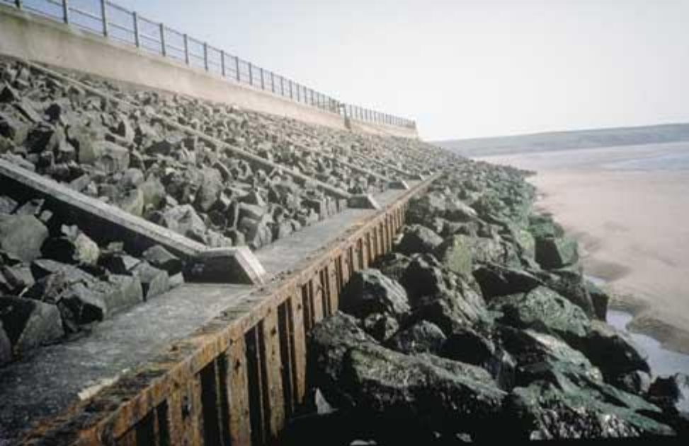
Rock faced concrete revetment
