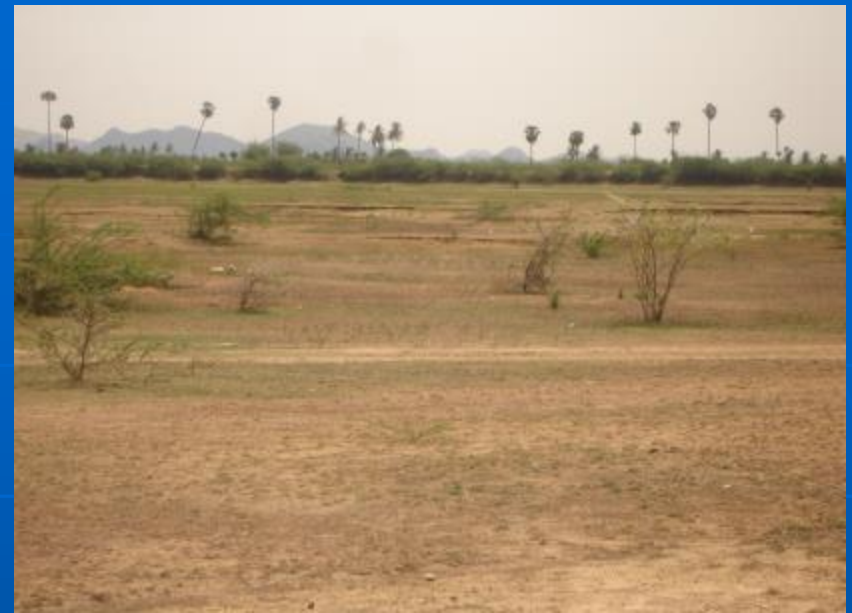
(2) TOTALLY DEFUNCT TANK
