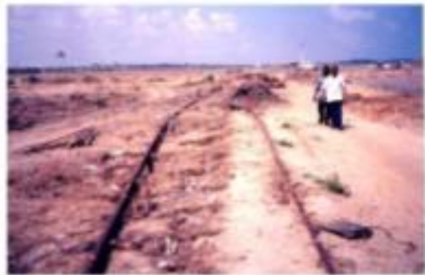
(E) Collapsed railway line - Nagore railway station
