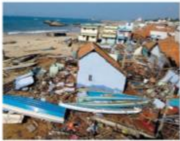
(A) Damaged houses - Pudukkuppam village
