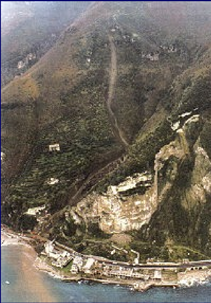
Pozzano (Castellammare di Stabia) – Italy. Landslide type: Debris flow
