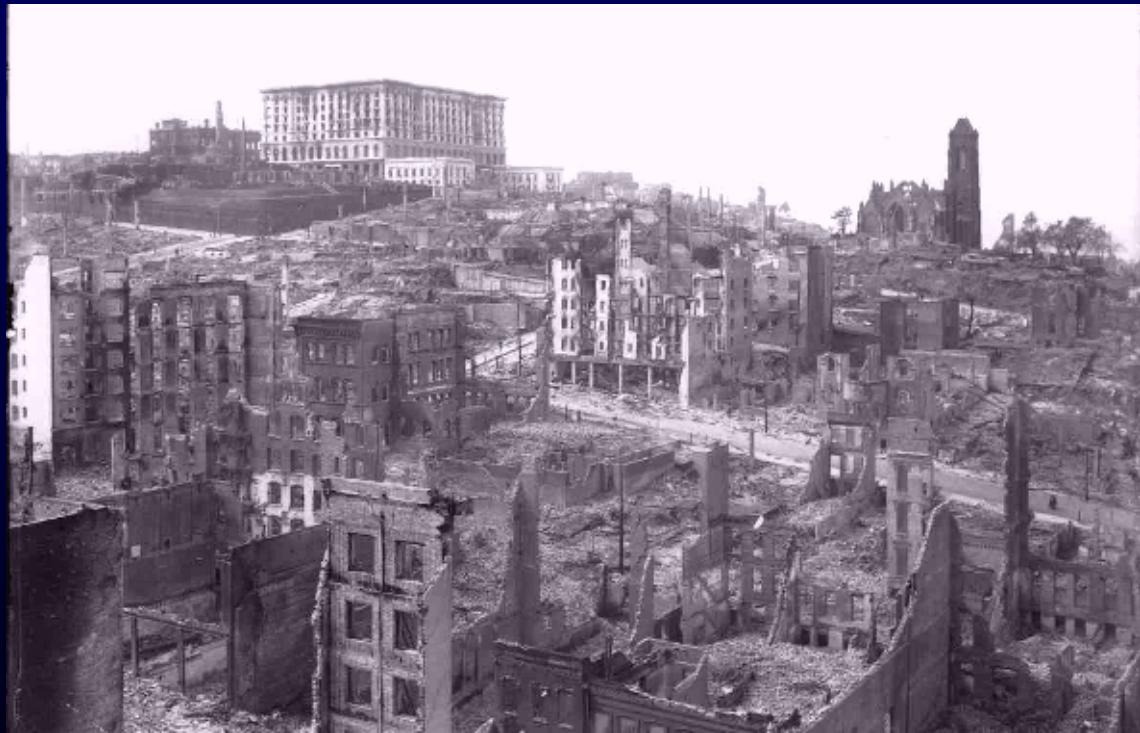
1906 San Francisco earthquake
