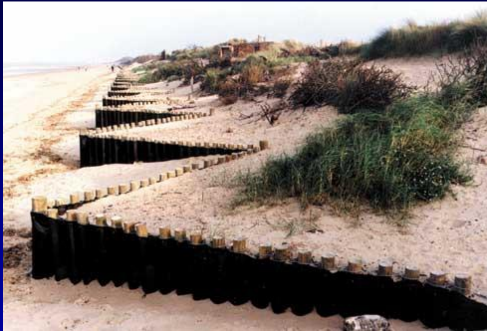
timber and geotextile
